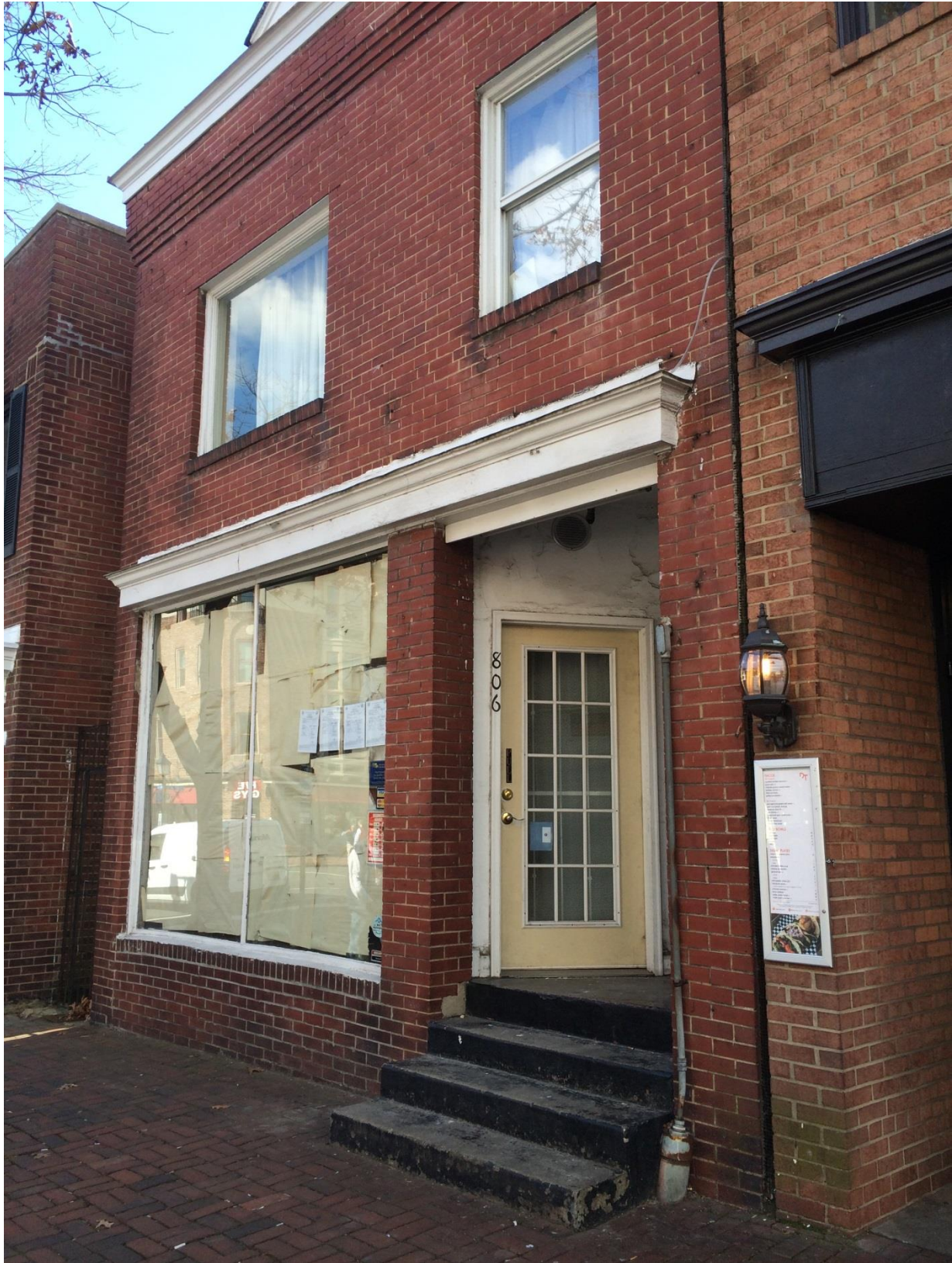
Figure 2: existing conditions at 806 King Street (photo taken January 2017). N.b. the 1936 design elements which were realized (including the fenestration with soldier-brick sills, corbelled brick cornice, and the first-story wooden cornice) in contrast to those elements that do not exist (including entrance pilasters, brick panels beneath the picture window, and the picture window's multi-light transom).
