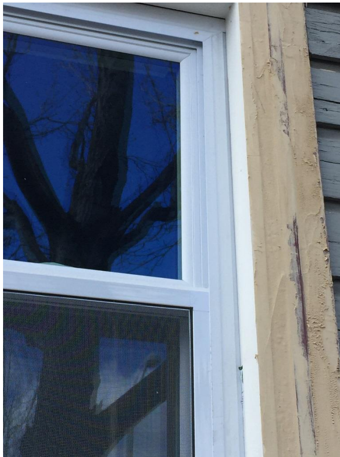
Figure 1. Detail of windows installed on front elevation without BAR approval.
