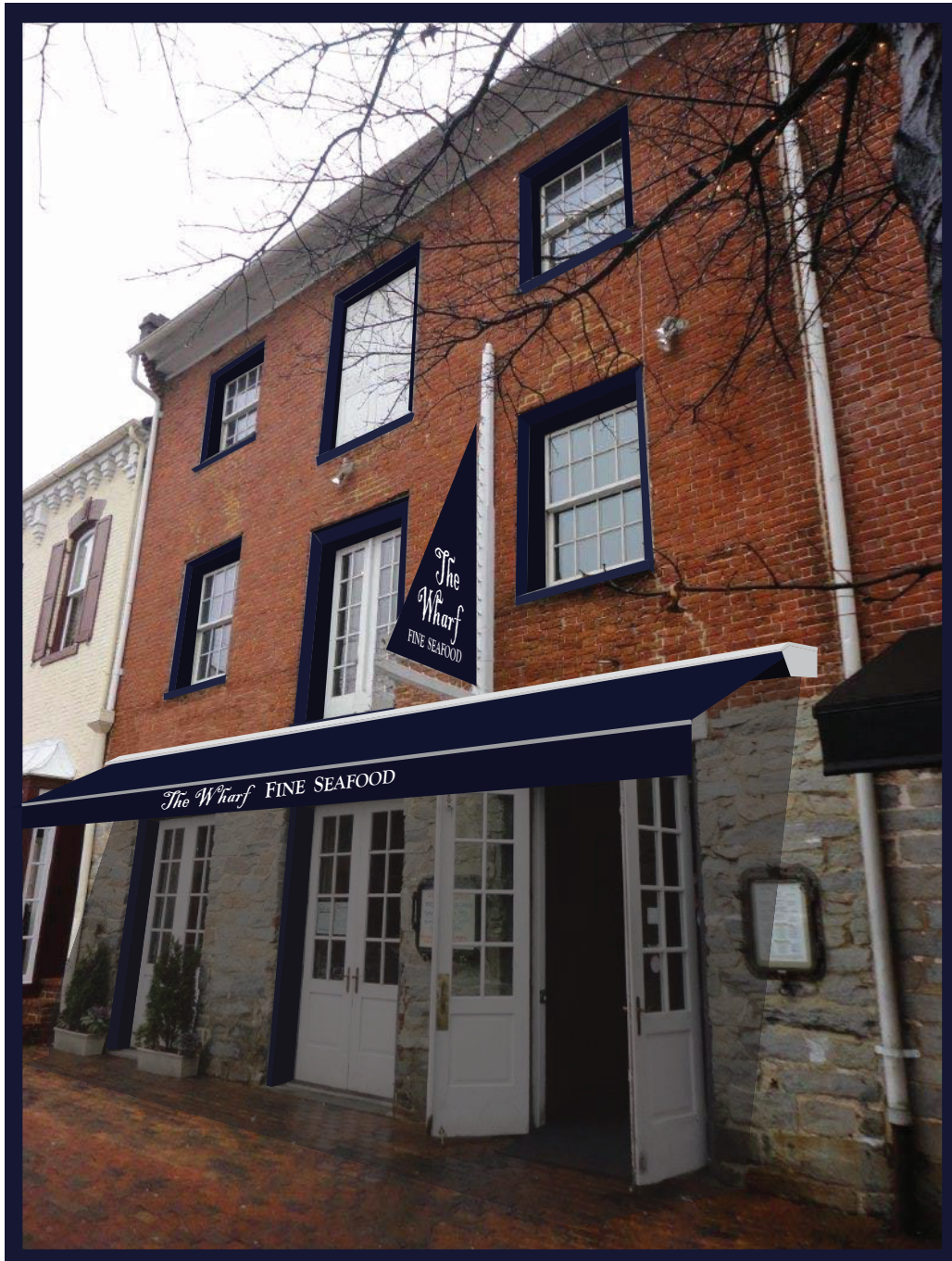
Retractable awning has an 8' clearance when fully extended to 5'-6" out
