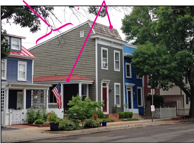
Roof materials can help differentiate between two periods of construction
