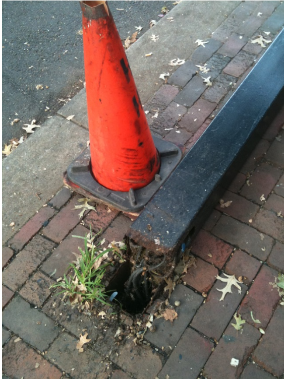
Figures 5 & 6: Rusty base and fallen Gadsby street light pole
