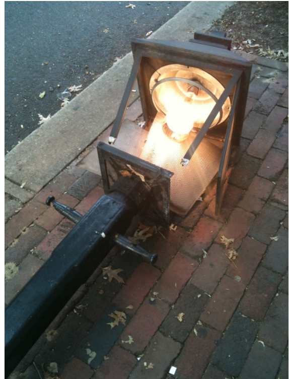
Figures 5 & 6: Rusty base and fallen Gadsby street light pole
