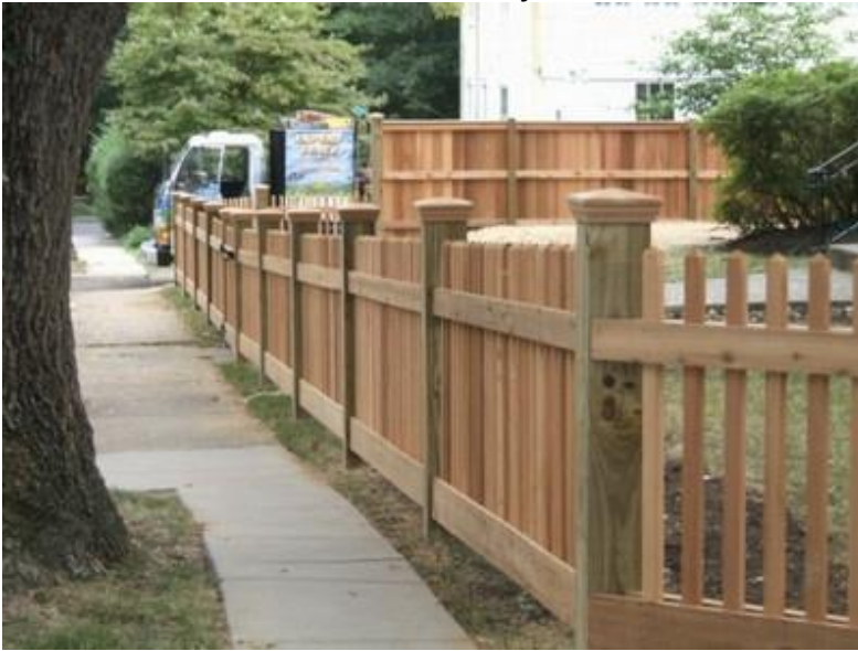
4' Cedar Picket Fence at front side yard location
