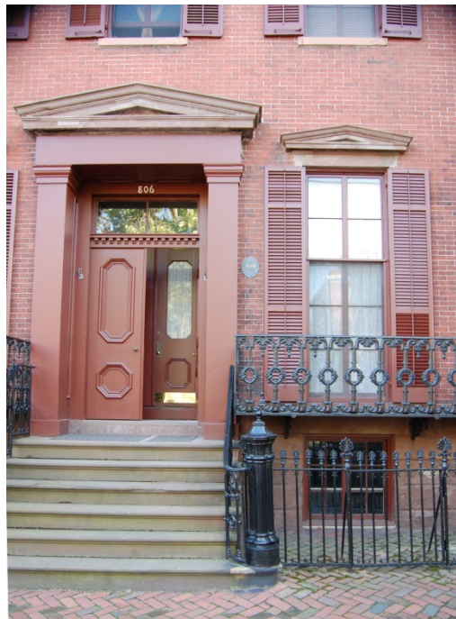
Figure 1: 806 Prince Street sandstone lintels
