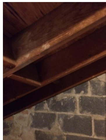
Figure 2: Photos of 20 th century framing: second floor ceiling joists and roof rafters
