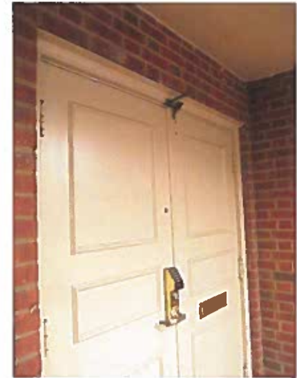
NEW DOORS TO HAVE SAME PANELING PATTERN AS THE EXISTING. ONE DOOR LEAF WILL BE WIDER THAN THE OTHER TO MEET ADA. DOORS WILL BE PAINTED TO MATCH EXISTING. HARDWARE TO MATCH EXISTING IN FINISHES AS WELL.
