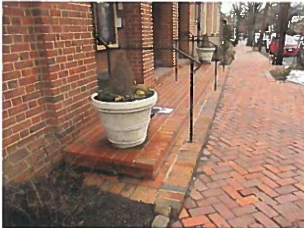
BRICK ON THE RAMP TO MATCH EXISTING AT THE TOP STEP IN COLOR AND SIZE AND PATTERN AS SHOWN ON PLAN.
