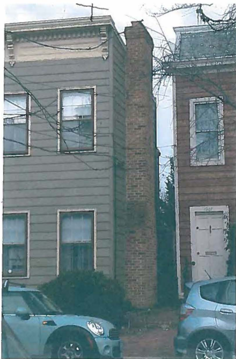
YARD BETWEEN 1209 & 1207 PRINCE ST NOTE ORIGINAL CORNICE AT 1209 PRINCE ST. - WINDOWS ALTERED & CHIMNEY ADDED C. 1971
