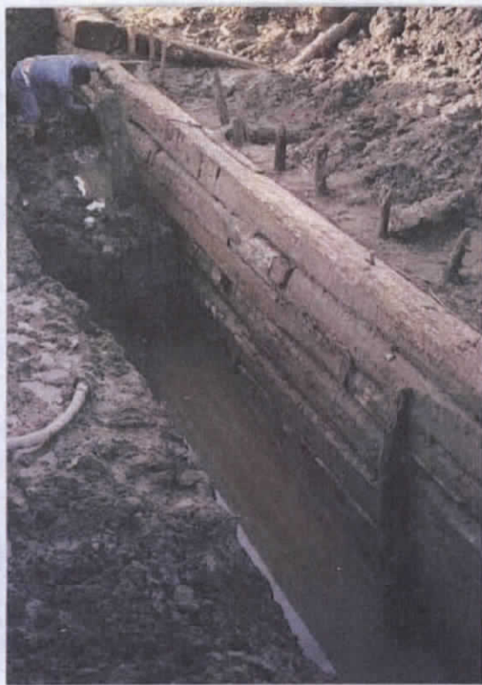
Figure 22: Keith's Wharf Bulkhead and Tie-Back Braces (Engineering Science 1993)
