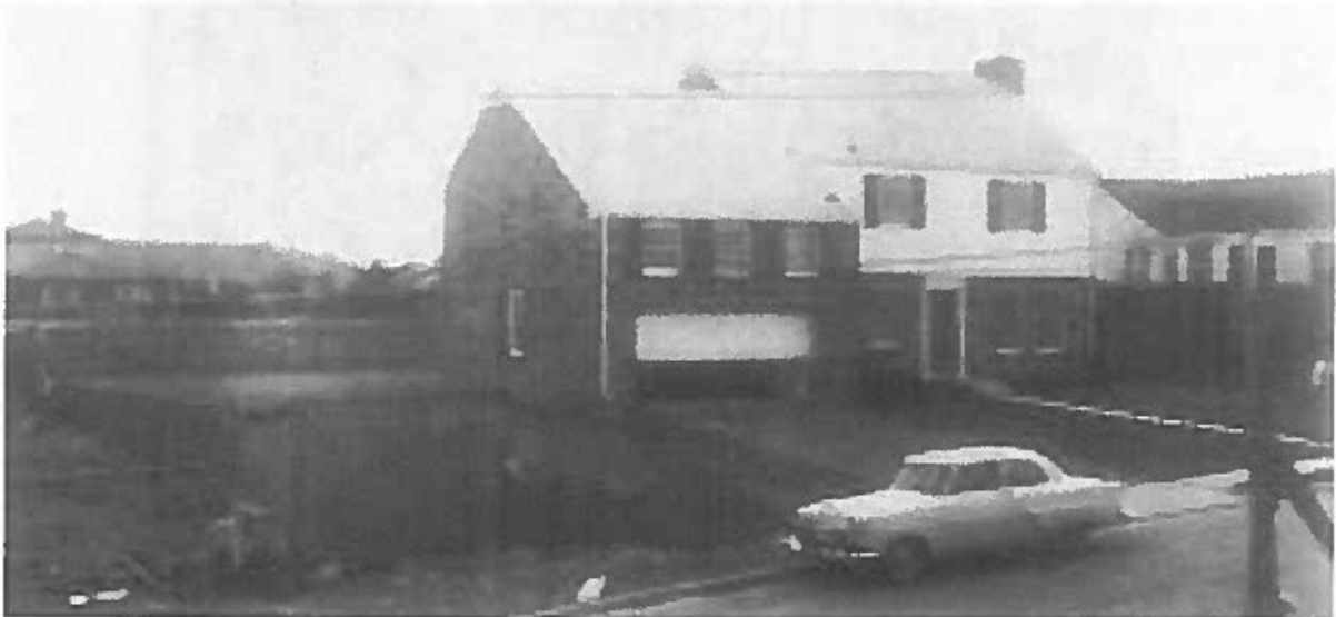
The Fords' house under construction in 1955 (National Park Service photo)
