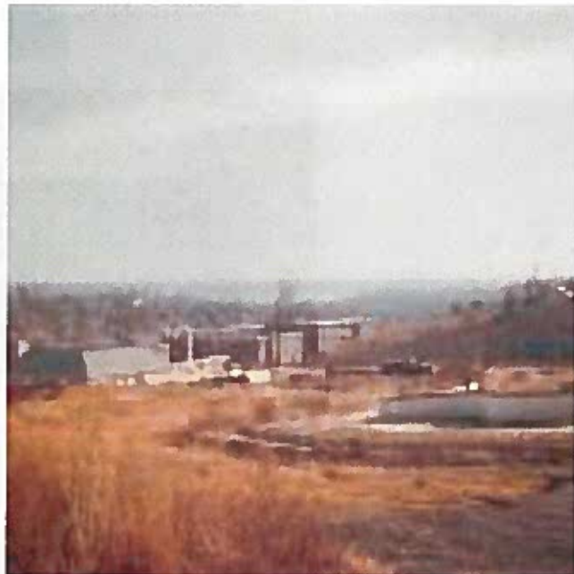
Beech's house at 812 Vassar Road under construction in 1956, showing "Beech's View" - the view he deliberately created for himself down to the Potomac River (courtesy Helen Baughman)
