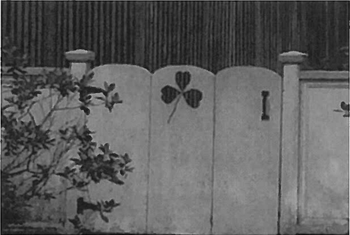
The original gates from the 1948 house of Rozier J. Beech, Clover's original developer
