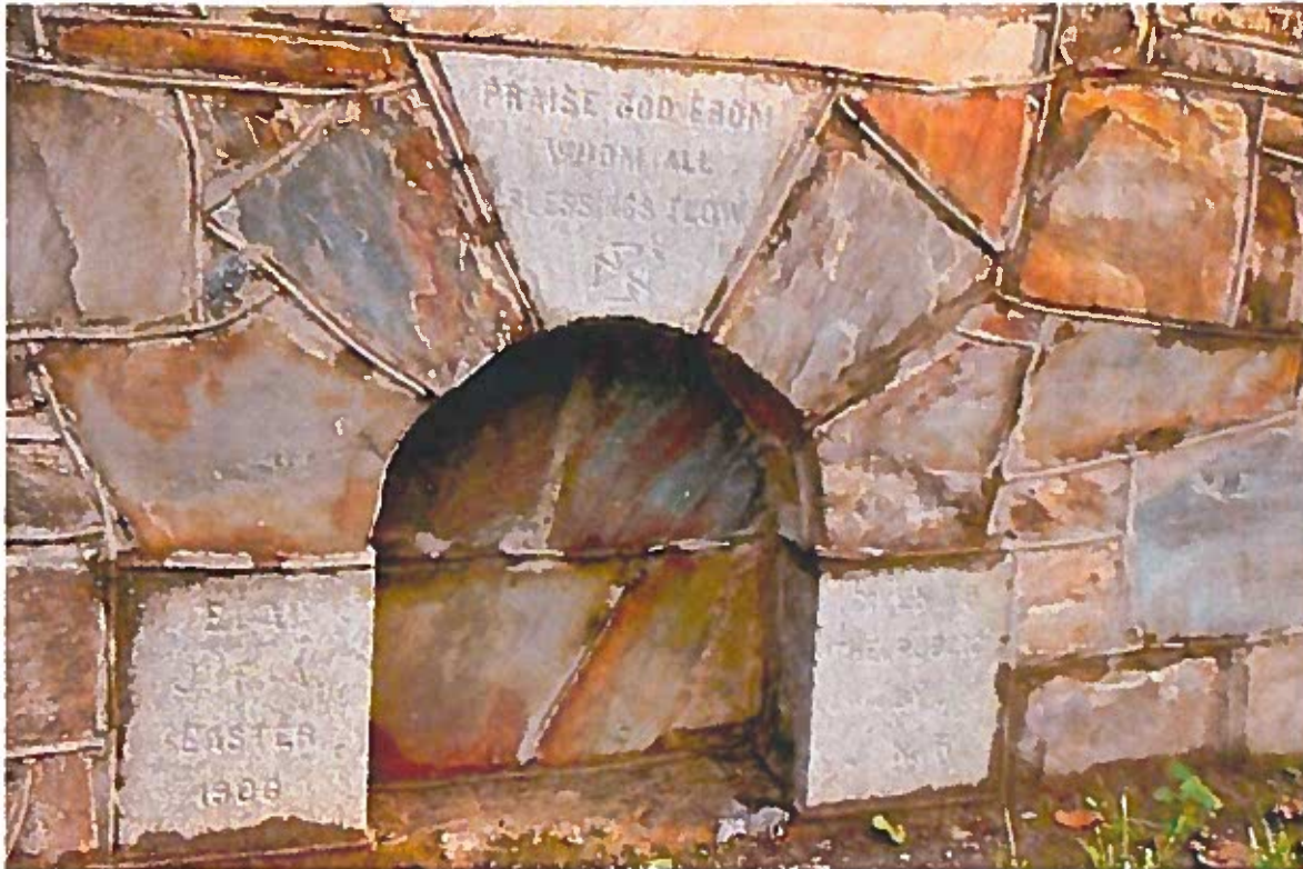
Niche in the wall at 810 Janneys Lane
