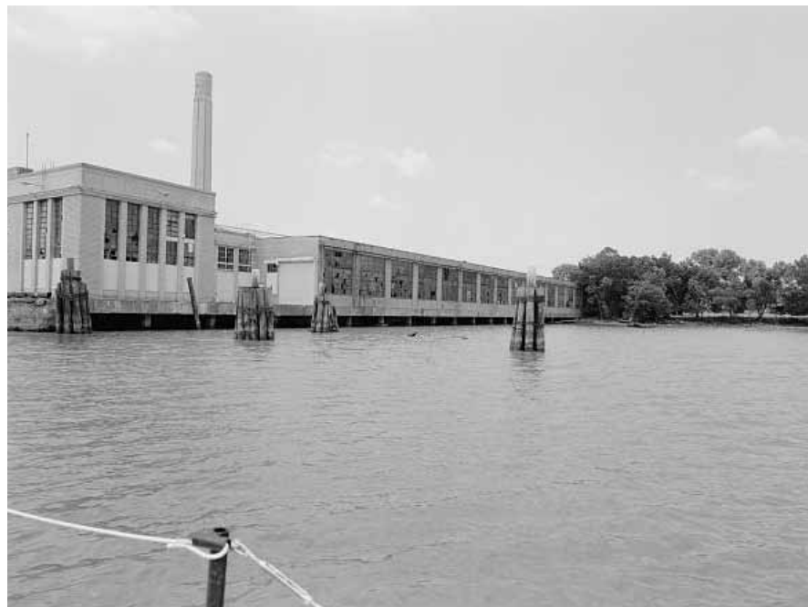
View of north elevation: With their different grid orientations, a hyphen connects the administration and assembly buildings. Each building façade expresses the functions within narrow window bays for offices in the administration building and larger glass filled square bays for the assembly building.
