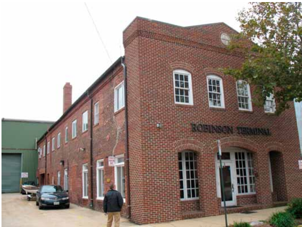
1-VIEW OF NORTH & EAST FAÇADES: The current street façade dates from the early 1990s. The original east façade openings have been heavily altered.
