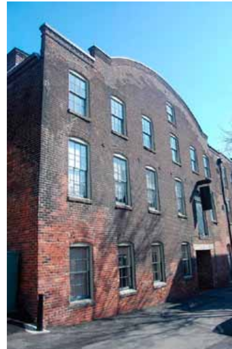
Crilley Warehouse at 216-220 North Lee Street, circa 1850, renovated 1970s: Note the segmental parapet wall extending above the structure's roof.
