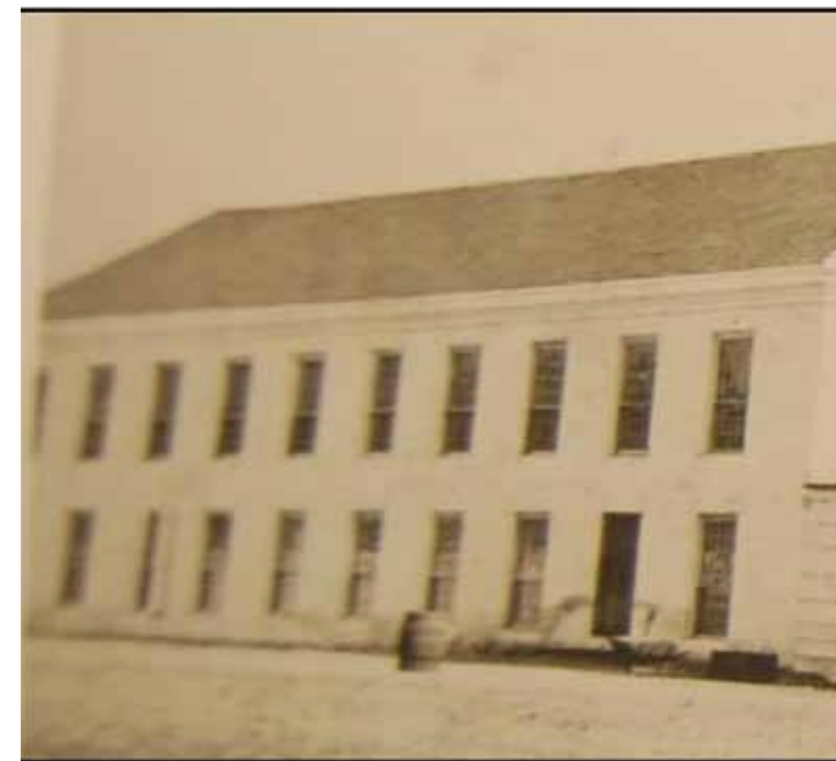
10-VIEW OF THE WEST ELEVATION OF THE COOPERS SHOP, circa 1864 (left) AND VIEW OF EXISTING BUILDING (right): The historic view shows that the second story windows were as large as the first story and had a straight header. Compare this with the segmental arched headers of the late 19th century building that replaced the earlier structure.
