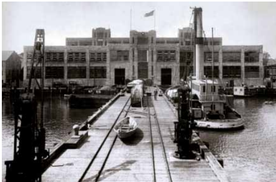
The Torpedo Factory in the 1920s (Library of Congress): The industrial aesthetic is clearly derived from the building's manufacturing functions with a rigid structural frame clad in a stucco cement, serving open floor plans with uniform large bays with extensive glass.
