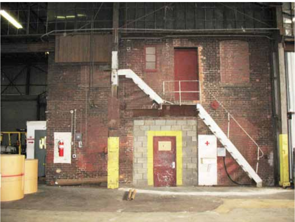
2-VIEW OF THE SOUTH FAÇADE: Encapsulated by later construction, this elevation has been extensively modified. Despite the changes, the original three bay configuration is evident upon close inspection.
