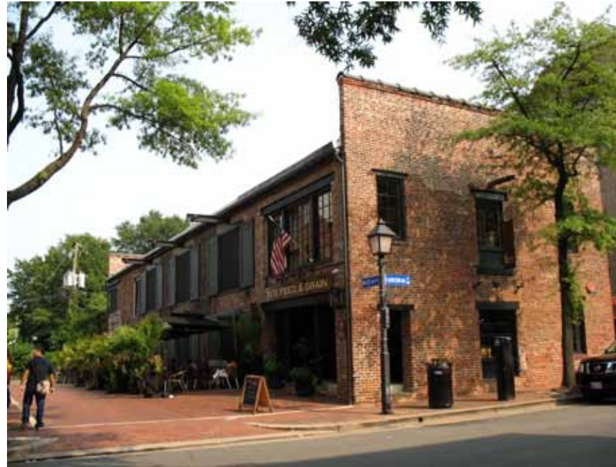
106 South Union Street, circa 1916: As an example of brick masonry common to many of the commercial/industrial structures, the range in color (medium red-orange), light mortar, and texture of the molded brick are defining characteristics. Note the extended parapet of the end wall. A recent adaptive re-use incorporates black multi-paned metal windows and large sliding doors with steel lintels.
