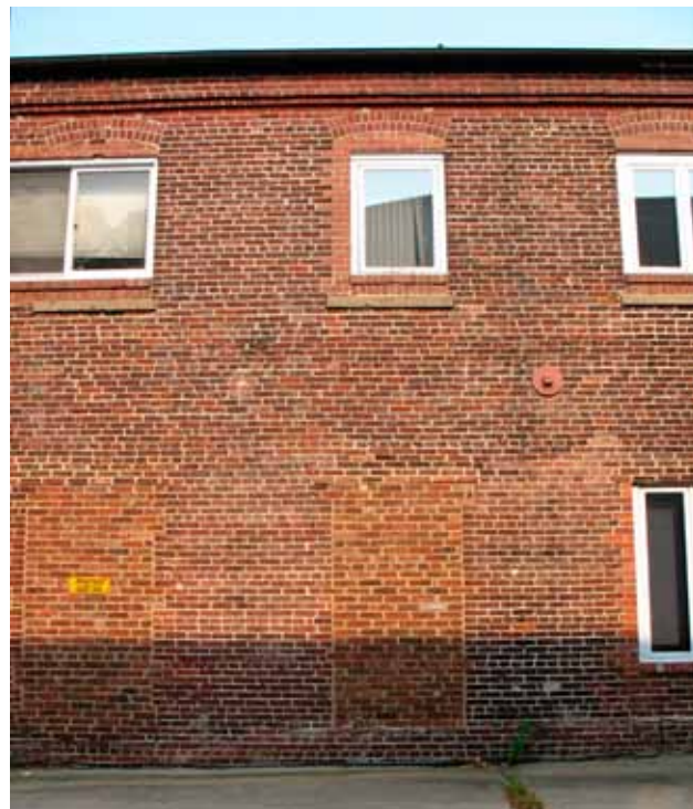
7-DETAIL AT WEST FAÇADE: Windows at the ground and second levels were originally aligned. Note the concrete sills.
