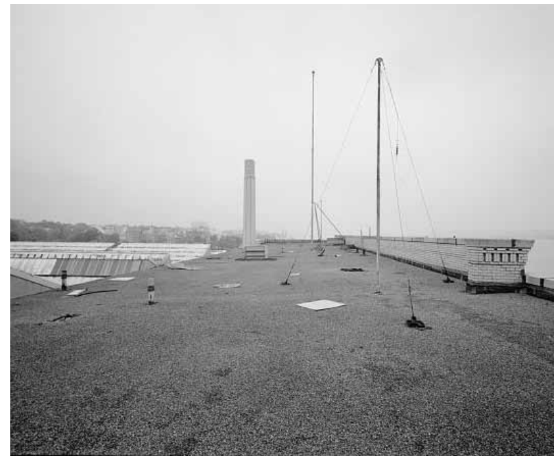
View of administration building's roof: A raised parapet along the center section screened the supporting structure for the Ford logo.
