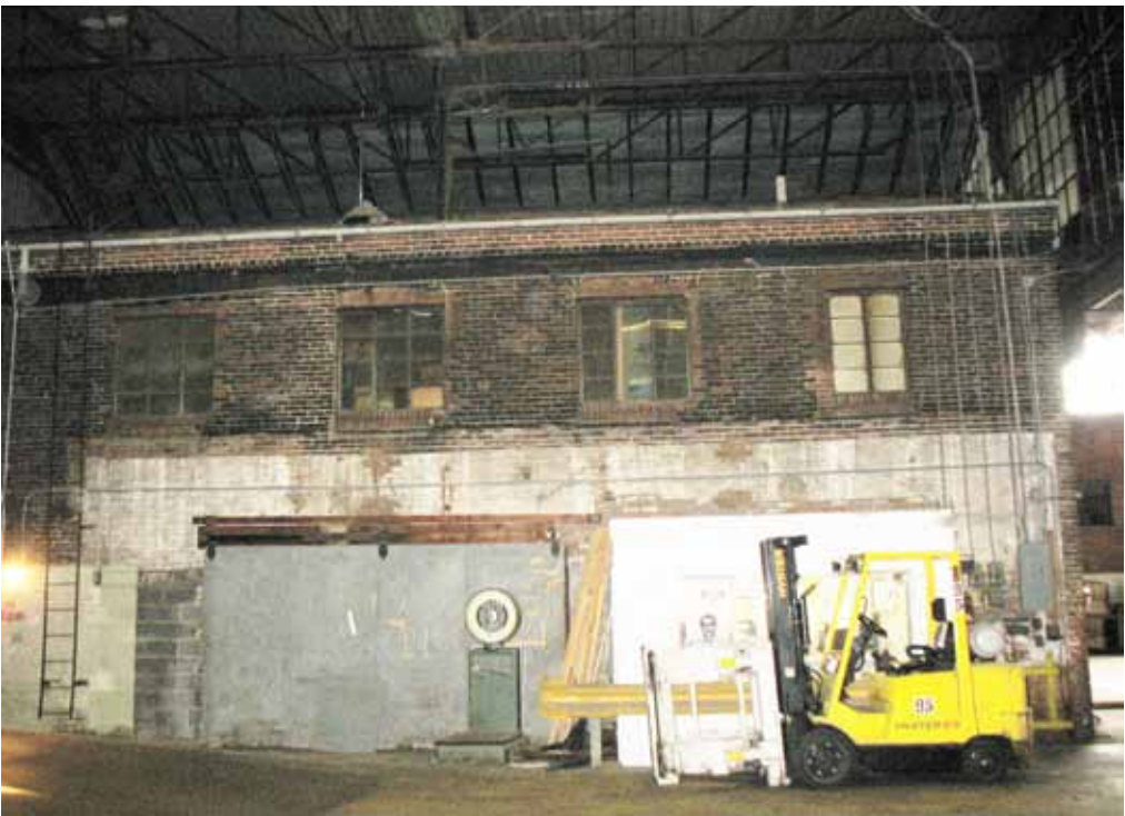
4-VIEW OF WEST FAÇADE: The portion of the west façade within the warehouse retains the outline in white of an earlier structure removed.
