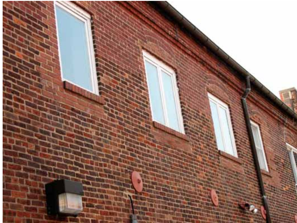
5-DETAIL AT EAST FAÇADE: Examination of the brickwork reveals the size and location of original narrower openings with segmental brick arched headers.
