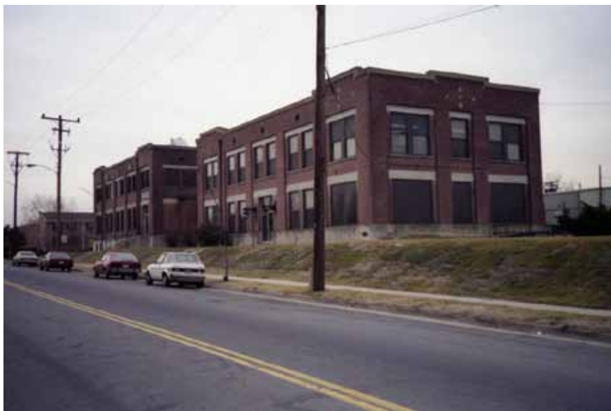
Santa Fe Railway Administration Building, early twentieth century (demolished): This pair of identical structures features 2-story bays with paired windows, 3 bays wide and 5 bays long. The double height reading is reinforced with brick spandrels and cast stone lintels. The end bays project slightly from the rectangular form as does the center bay at each end.
