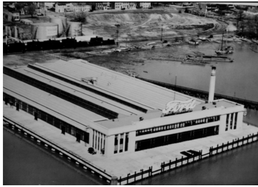
Ford Assembly Plant, Alexandria, circa 1930, Aerial View: Built on a platform supported on piles, the building is comprised of two elements, the administration building fronting the water and the assembly building behind it. Each was built with a different orientation of their planning grids. The administration building aligned with Alexandria's street grid while the assembly building was oriented to the river channel. Note the high contrast between the yellow brick masonry and the dark window bays.
