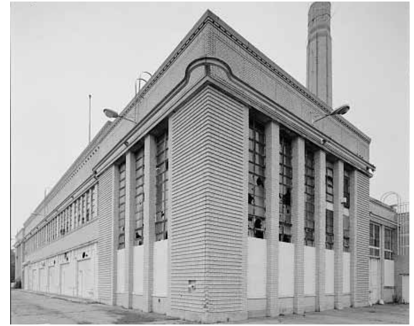
View of northeast corner of the administration building: The administration building's river facade is composed of a raised center section with a horizontal emphasis, flanked with matching end pavilions. The pavilions featured highly articulated brick detailing at corner piers and entablature. The vertical expression of narrow multi-story bays was a counterpoint to the horizontality of the center section.
