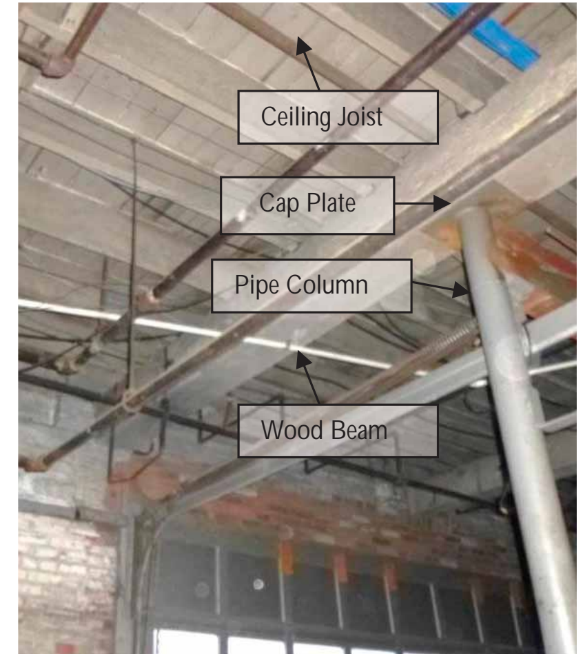
Interior Floor Framing
