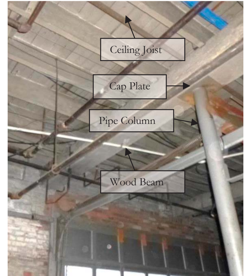
Interior Floor Framing
