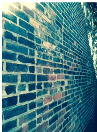
Infill Ghosting – South Elevation
