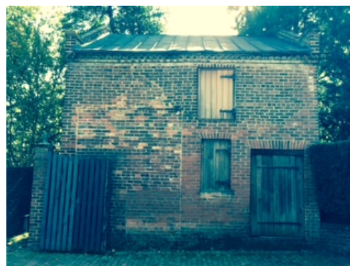
Infill Ghosting – North Elevation; All windows and doors have metal lintels - indicating at a minimum a repair to the opening.
