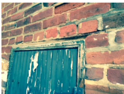
Metal Lintel above door – East Elevation
