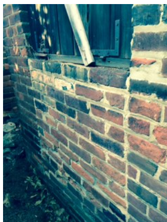
Infill Ghosting Below window on South Elevation
