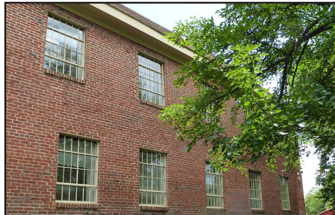
Detail of West Side of Historic Mill
