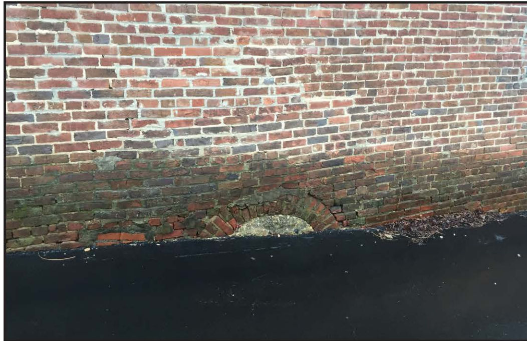
Location of Grist Mill Axle Entry Point on West Face
