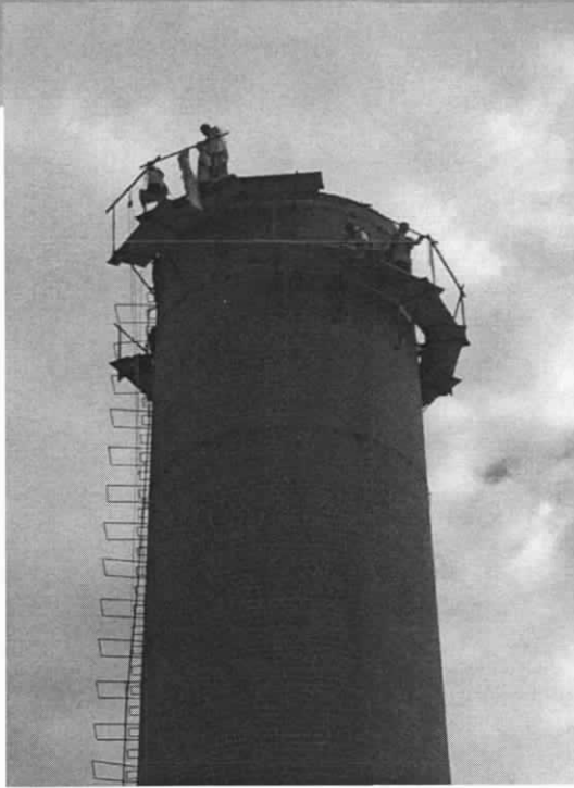
Workers demolishing the stack from the outside
