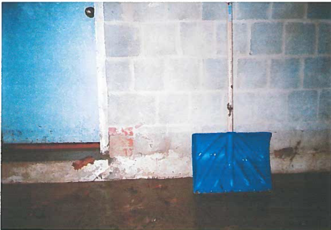
Flood water ran beneath door into basement level – note water level line on wall
