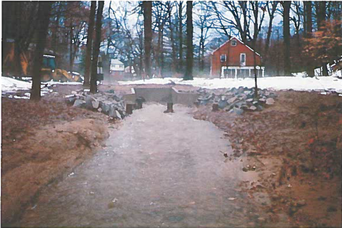
Upstream view - Water receding – line between snow and dirt indicates flood level
