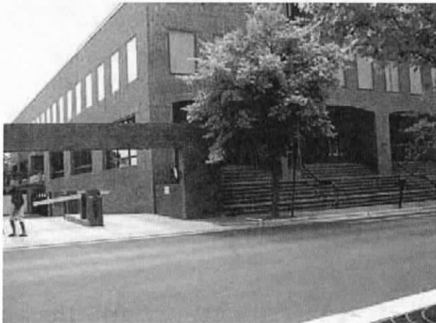
6A: Commercial space above parking garage. First floor elevation at 11.6 ft. No flood protection is needed as the structure is above the garage.
