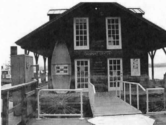
6B: Alexandria Seaport Foundation located along the water. May need some flood proofing options for the boat building and their office.
