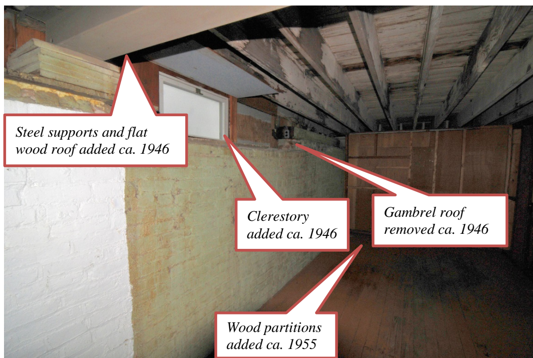
Figure 21. Interior of east elevation of 226 The Strand, showing where brick was removed unevenly to create a flat roof (2015).
