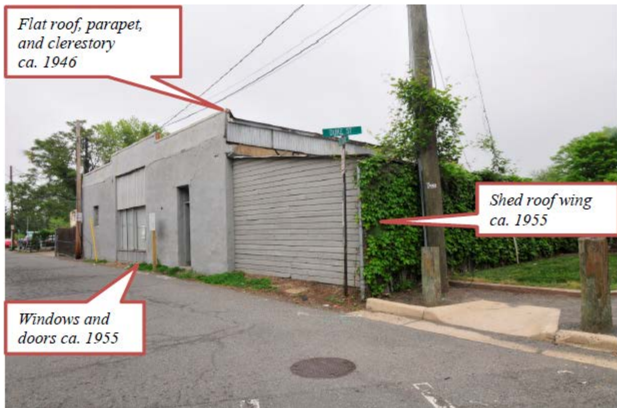
Figure 1. Street view of 226 The Strand, identifying some key building elements and date of construction (from applicant's history report prepared by Thunderbird Archeology).
