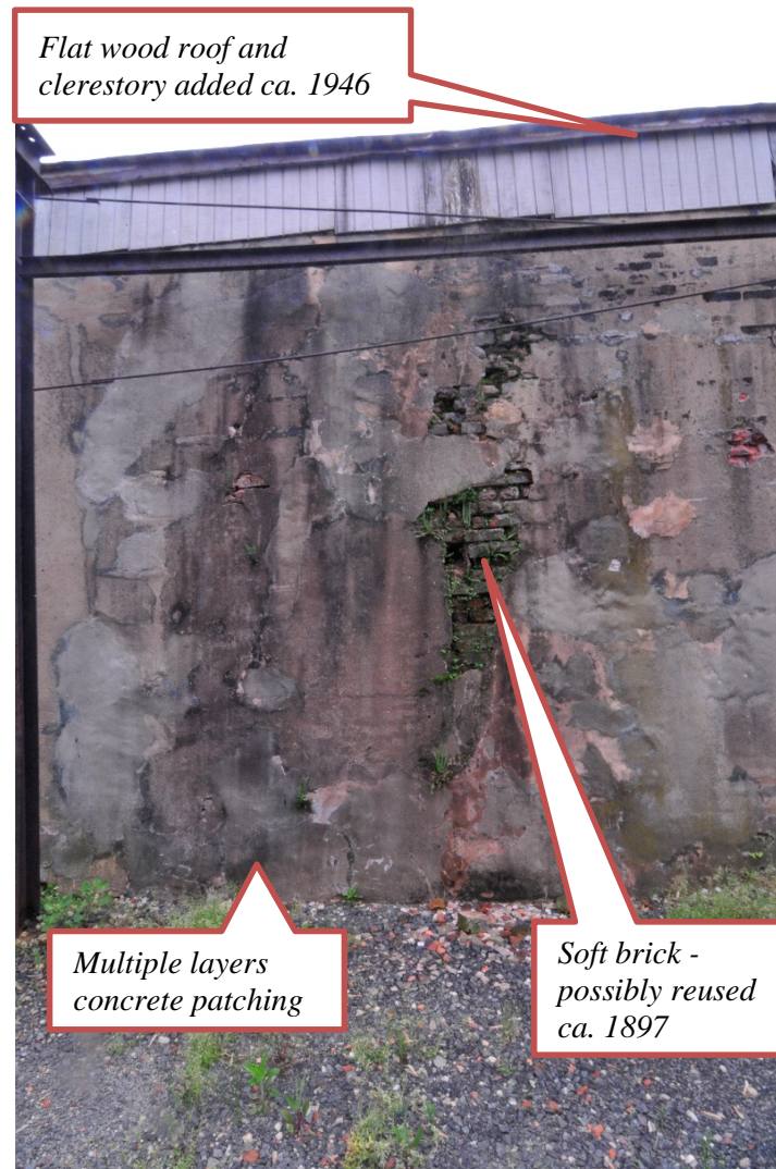
Figure 24. North elevation of 226 The Strand, showing altered roof line, buckling of brick and multiple layers of deteriorating concrete patching (2015).
