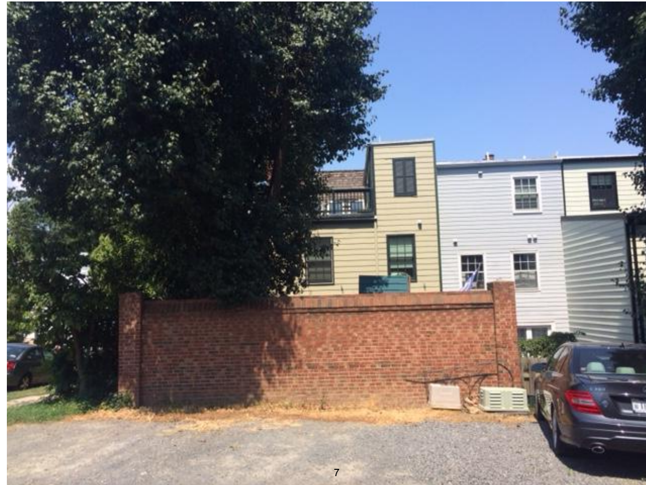
VIEW C - FROM ALLEY DIRECTLY BEHIND HOUSE. APPROXIMATELY 45 FEET FROM REAR OF HOUSE
