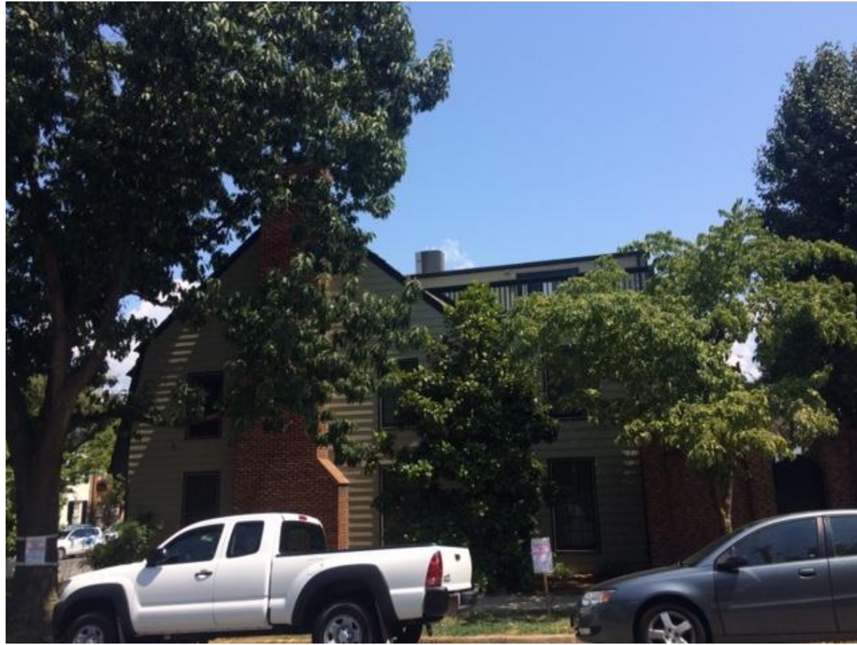
VIEW A - FROM ACROSS COLUMBUS STREET DIRECTLY ACROSS FROM SIDE OF HOUSE. APPROXIMATELY 45 FEET FROM SIDE OF HOUSE.
