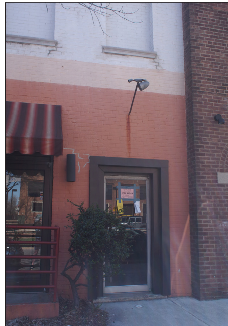
existing brick painted - proposal to repaint brick, excluding any existing stonework
