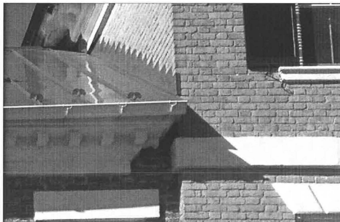
Detail of south wing cornice and roof abutting the south wall of 201 S. Lee Street.
