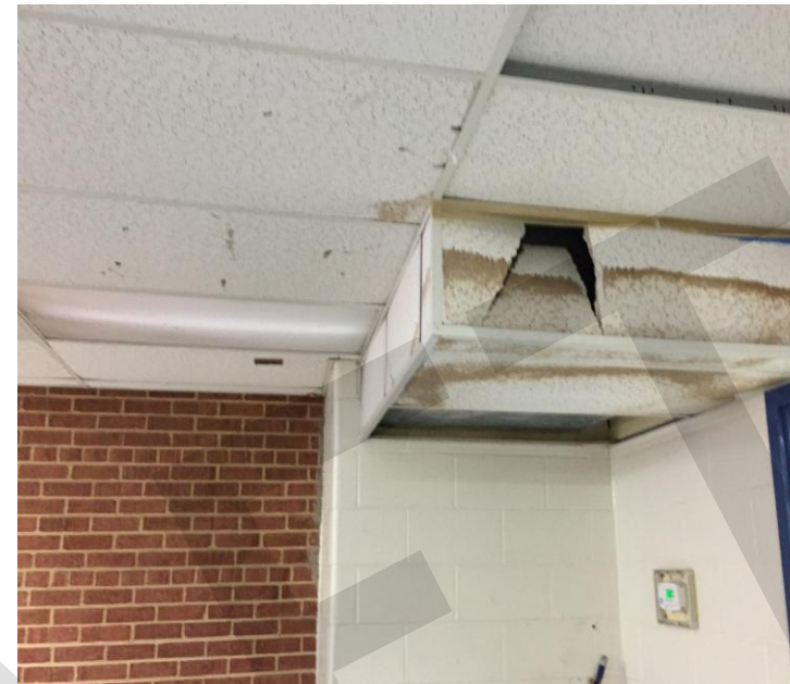
DETERIORATION OF MP-ROOM CEILING
