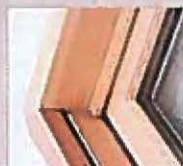
Traditional head with removable head parting stop
