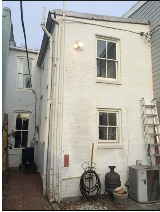
Figure 1: View of the east wall of 214 S Alfred St. The windows on the east elevation lack the jack arches of those on the south side of the ell and the modern brick infill on the lower level reflects an earlier addition.
