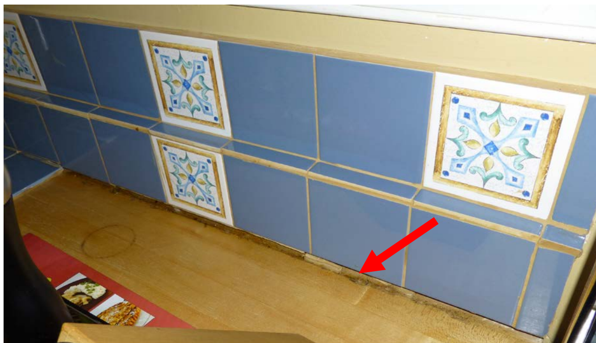
Figure 5: Evidence of settlement that is likely the result of rotted floor joists in close proximity to the earth below shown where the kitchen counter is pulling away from the tiled backsplash.
