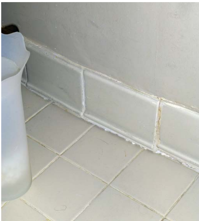
Figure 4: Weakened floor joists caused by previously leaking plumbing fixtures are likely causing the upstairs bathroom fixtures to sink, pulling the tile down and away from the wall.
