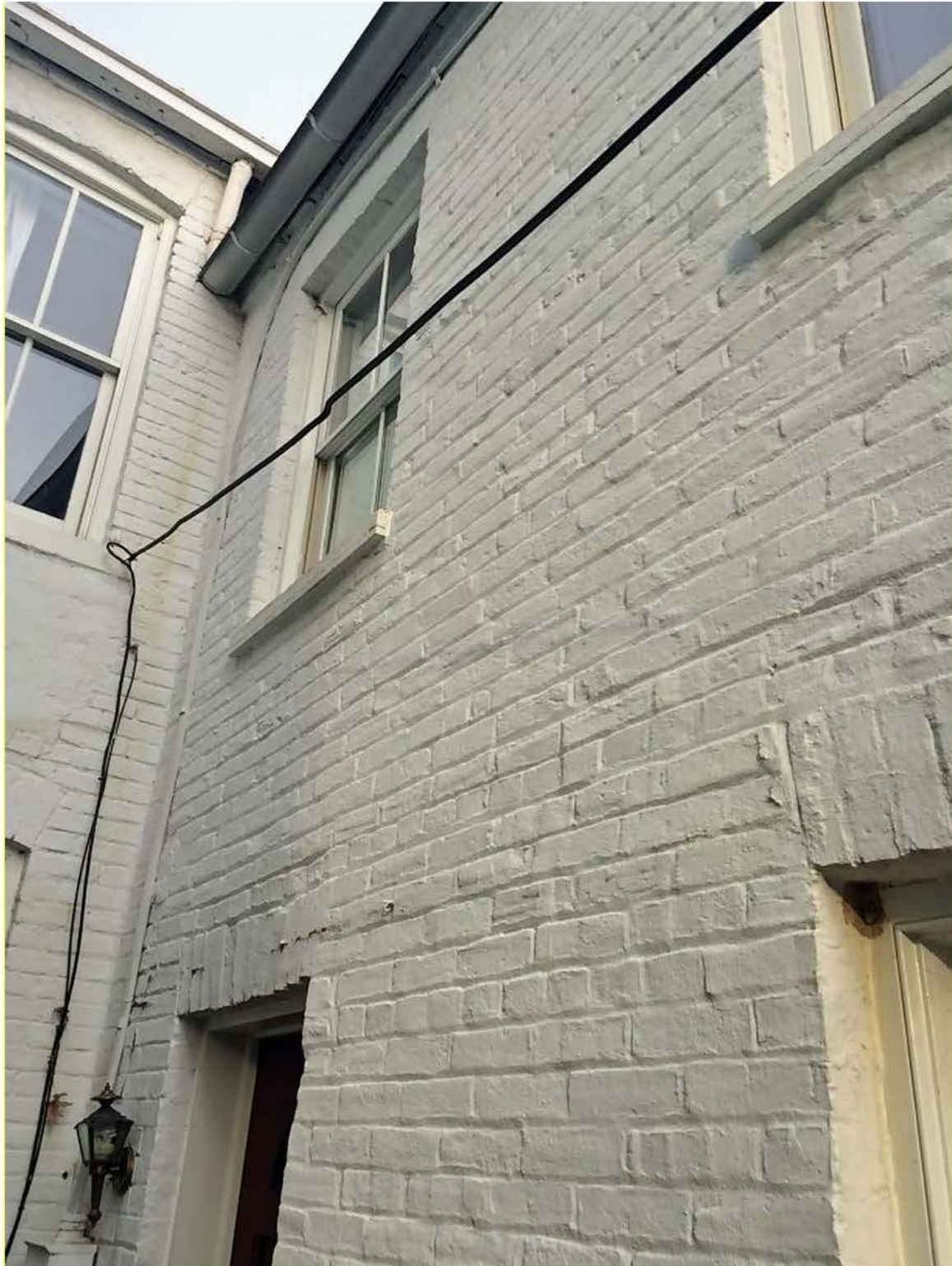
Figure 3: Condition of the south wall, which staff recommends be preserved. The inappropriate mortar repairs were likely a response to water damage – perhaps caused by previously broken or missing gutters above or rising damp from below.
