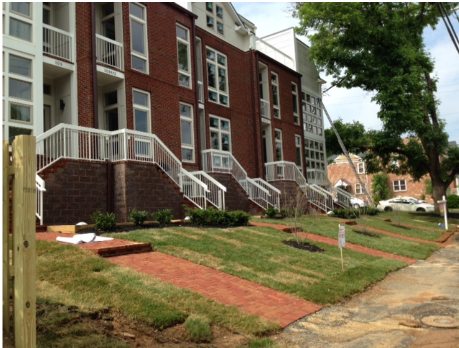
As built condition illustrating steeper lead walk grades to the front
