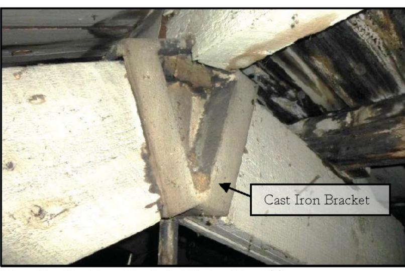
Figure 7 – Cast Iron Bracket at Peak of Roof Trusses
