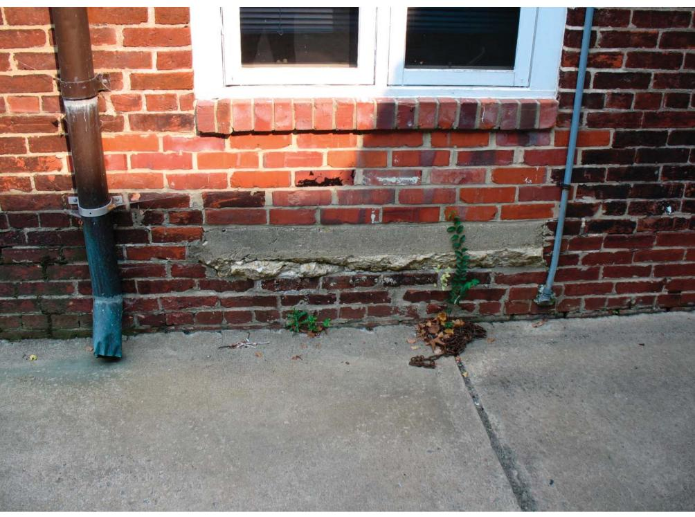
8-DETAIL AT WEST FAÇADE: Brick rolock sills were used when sills were raised.
