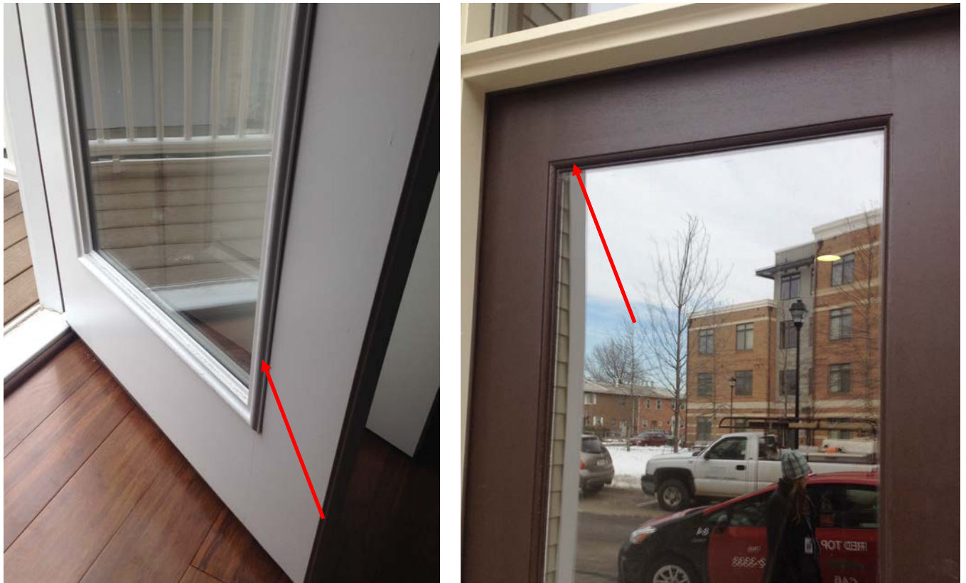
Figure 3. Left: Fiberglass door with raised sticking where glass meets rails and stiles. Right: Wood door with flush sticking where glass meets wood.
