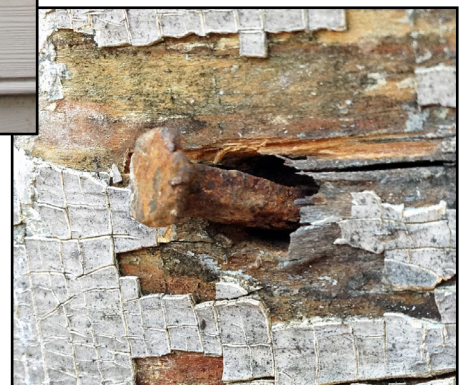
The investigation reveals an older layer of siding underneath.
