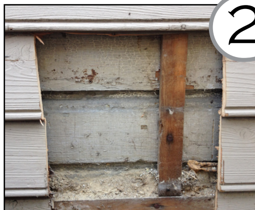
The investigation reveals an older layer of siding underneath.
