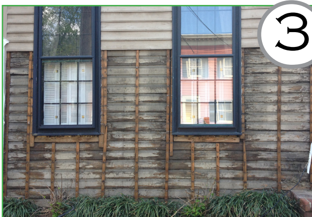
The contractor exposes more of the historic siding for staff to assess its condition. In this case, the historic siding is in very good condition and will be stripped and painted for re-use on this building.
