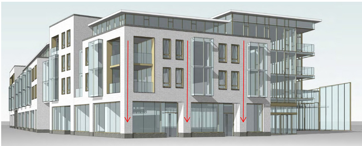
Figure 2: Red arrows in the present proposal show the load path traveling directly to the ground, a character-defining feature of Alexandria's historic masonry architecture, with large storefront windows below each bay
