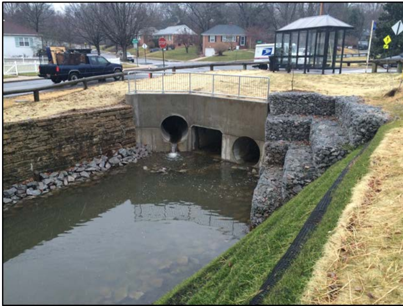
Newly constructed headwalls and channel improvements
