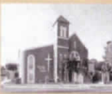
The Oakland Baptist Church on King Street, pictured after its 1928 construction, continues to serve the African American community. It represents the strength and durability of early church founders and descendants families, many of whom still live in the area. The church is listed in "The Black Book, African Church, and Home by the Spirit's Power."
