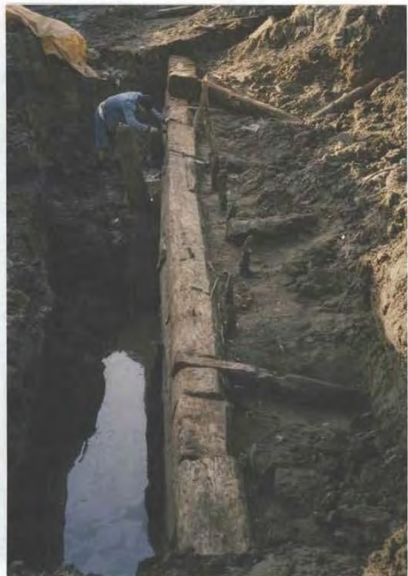
Exhibit 16: Keith's Wharf Bulkhead and Tie-Back Braces (Engineering Science 1993)
