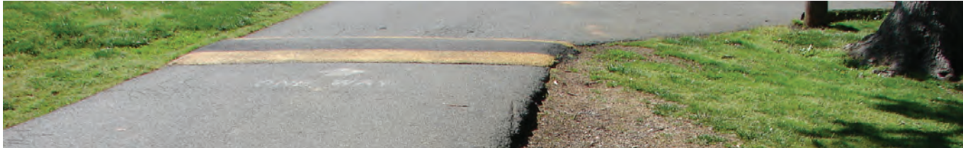
Figure 10 - Speed bump on paved loop path that does not meet current ADA standards
