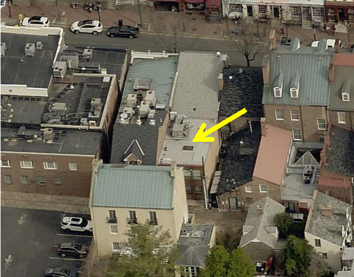
Figure 2: Arrow shows the current condition of the rooftop at 212 King Street.
