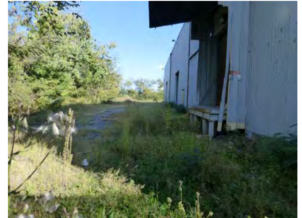
Original terminus of railroad tracks (north edge of site)
