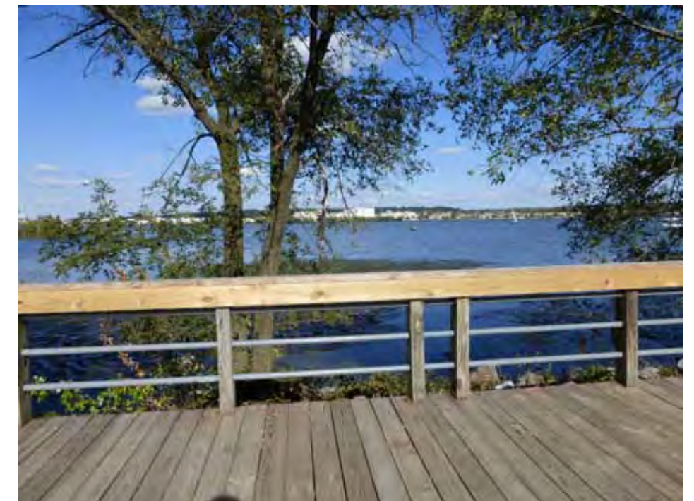
Railing detail looking north at edge of Oronoco Bay Park
