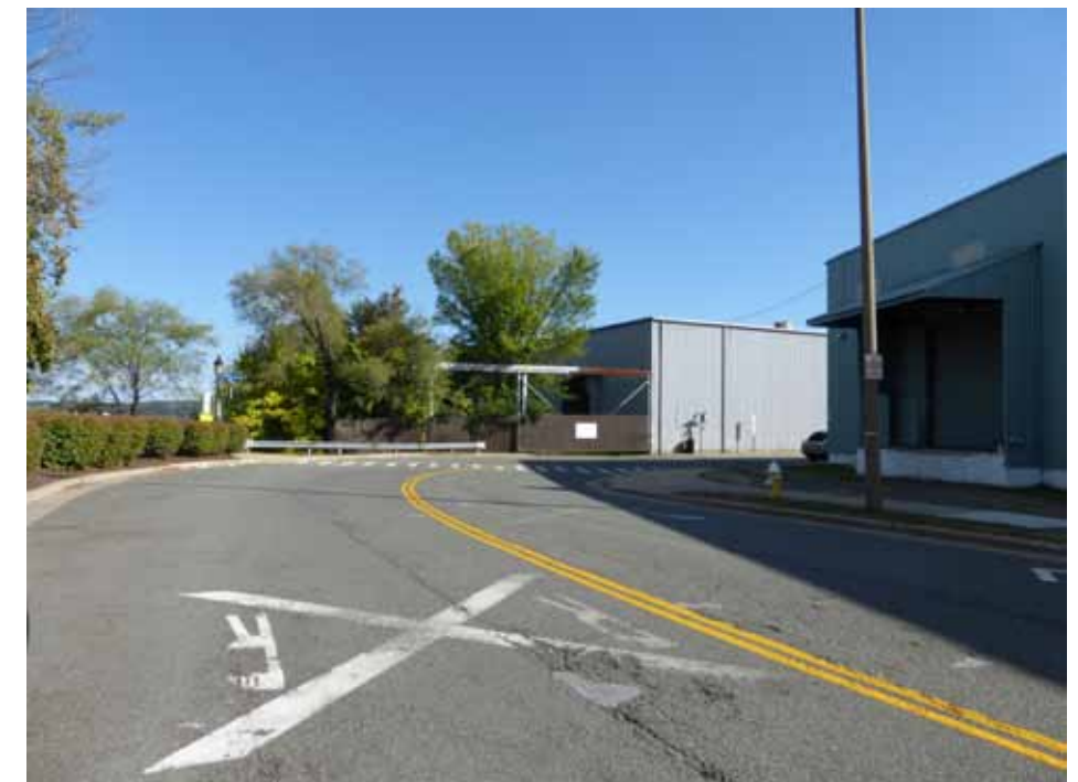
Railing tracks along north edge of the west warehouse
