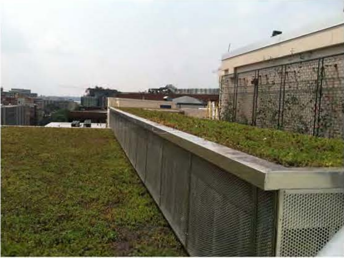
GREEN ROOF DUCT ENCLOSURE
