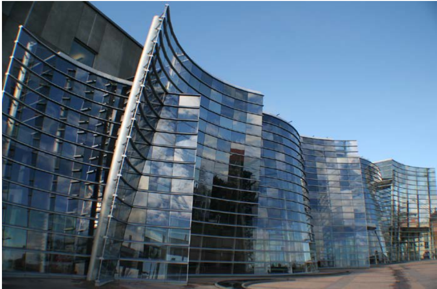
Figure 16: Potential design precedent for a sculptural, artistic, and creative pavilion facing the water. This design achieves its drama through the use of materials and the geometry of the walls, and does not depend on a roof form for expression. This is an image of the Christchurch Art Gallery in New Zealand.
