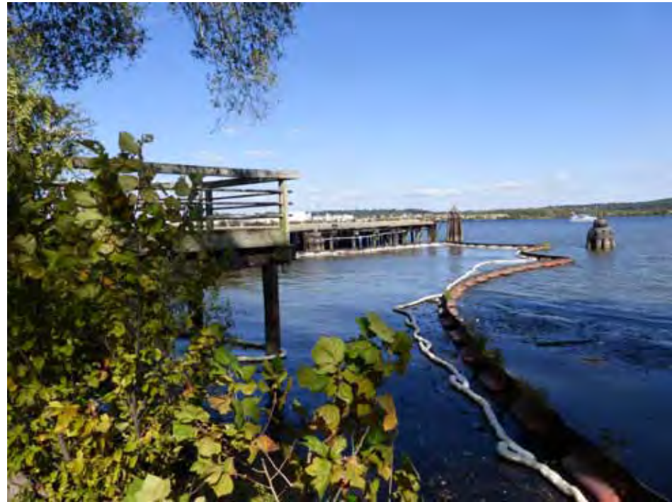
Existing West's Point Wharf
