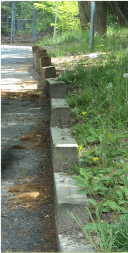
TIMBER RETAINING WALL UNDER PRESSURE (T-II-D)
