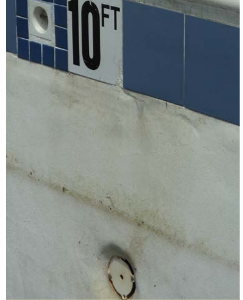
CRACKING POOL TILE (T-I-D AND T-III-A)
