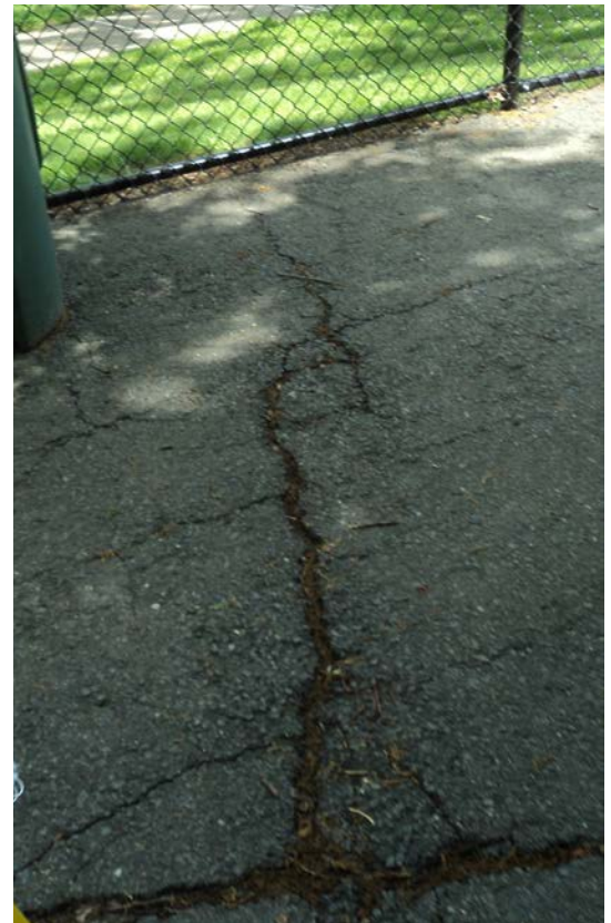
FAILING ASPHALT ENTRANCE (T-II-C)
