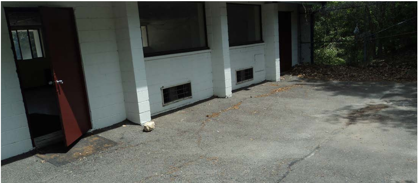
ASPHALT AT UPPER LEVEL ENTRANCE - CRACKING AND SLOPE ISSUES PRESENT (T-II-C)
