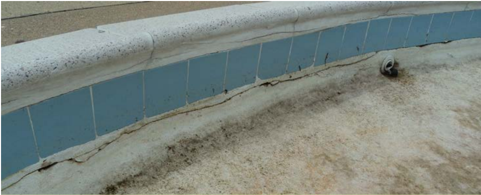
CONSISTENT CRACK AT WADING POOL (T-III-B)
