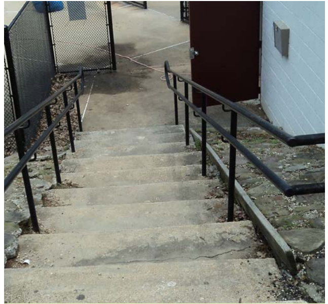
FAILING CONCRETE STAIRS (T-I-C AND RECOMMENDED T-III-C)
