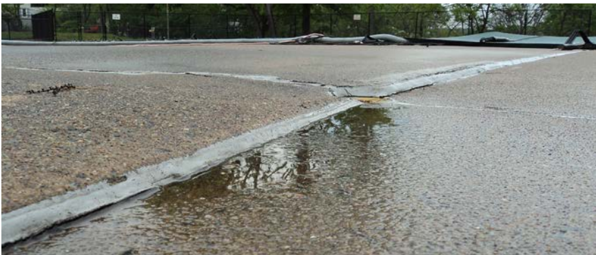
FAILING AND DAMAGED CONCRETE JOINTS (T-I-D)
