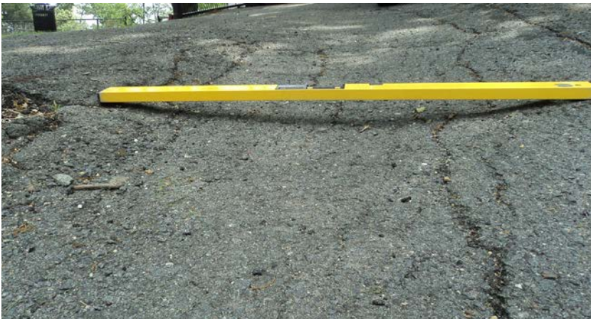
FAILING ASPHALT ENTRANCE (T-II-C). SEVERE SETTLING AND SHIFTING
