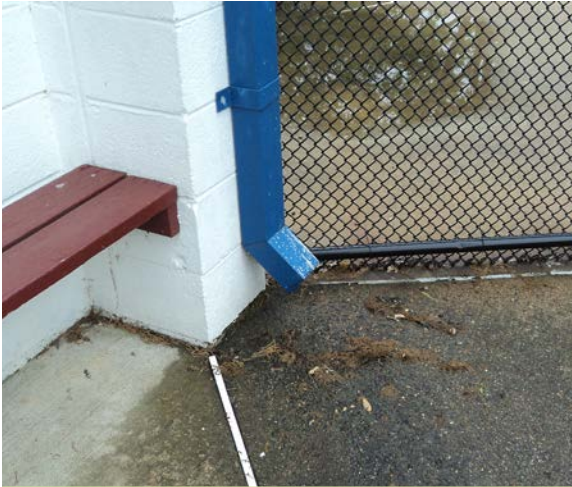
ROOF LEADERS AT POOL DECK WITH NO GROUND LEVEL CONNECTIONS (T-II-B)
