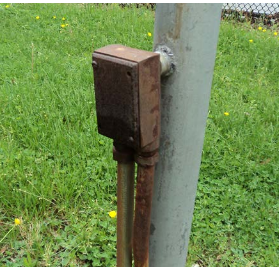
AGING LIGHTING EQUIPMENT - NO SEALS (T-II-F)
