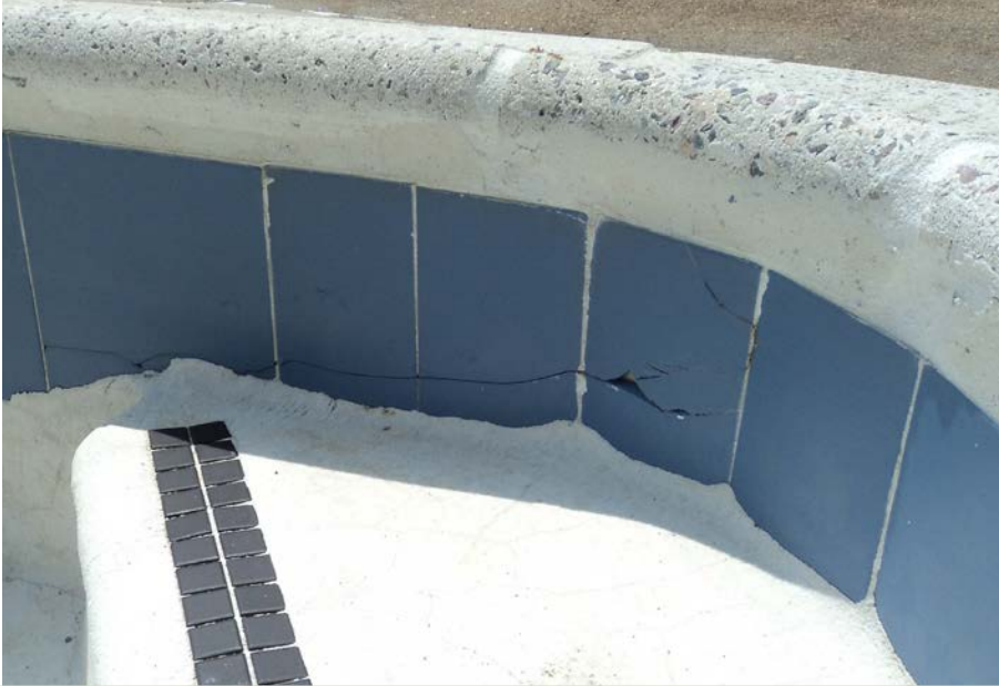
CRACKING POOL TILE (T-I-D AND T-III-A)
