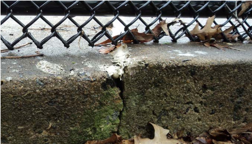
FAILING CONCRETE POOL DECK (T-II-A)
