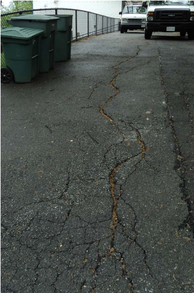
FAILING ASPHALT ENTRANCE (T-II-C)
