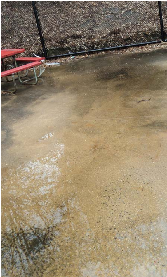
STANDING WATER - CLOGGED POOL DECK DRAINS (T-I-B)
