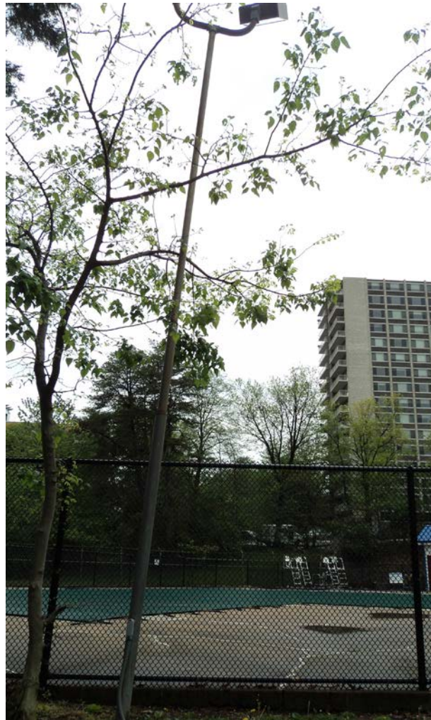
LEANING LIGHT POLE ALONG NORTH FENCE LINE (T-II-F)
