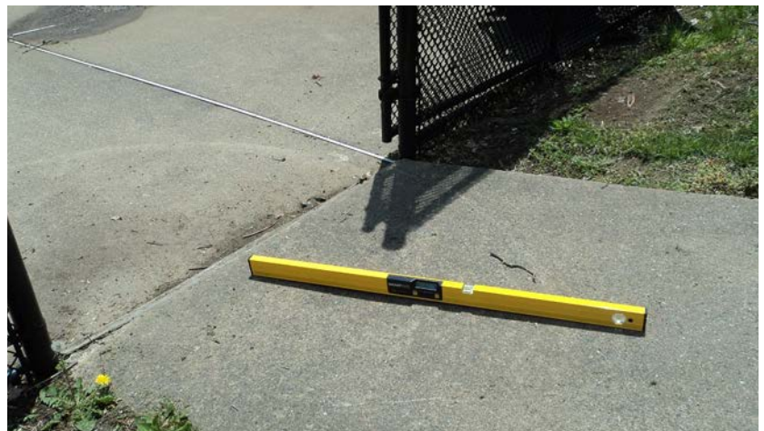
CONCRETE SIDEWALK TRIPPING HAZARD AND EXCESSIVE SLOPE AT WADING POOL ENTRANCE AND CONNECTION (T-I-A)
