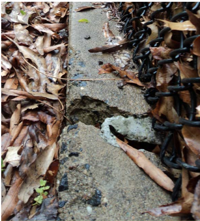
FAILING CONCRETE POOL DECK (T-II-A)
