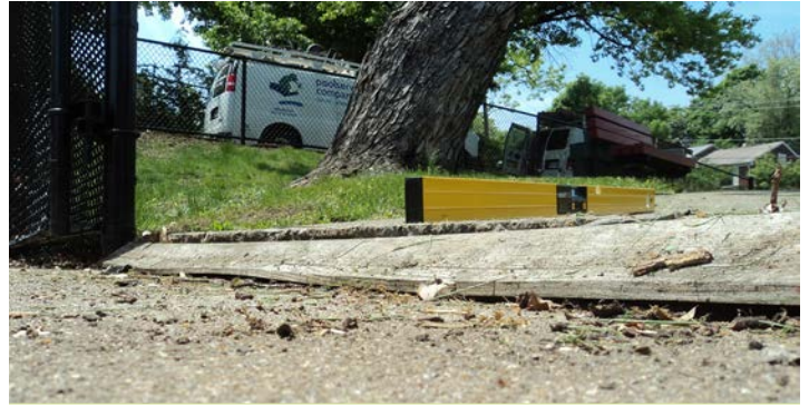
TRIPPING HAZARD AT CONCRETE SIDEWALK ENTRANCE TO WADING POOL (T-I-A)
