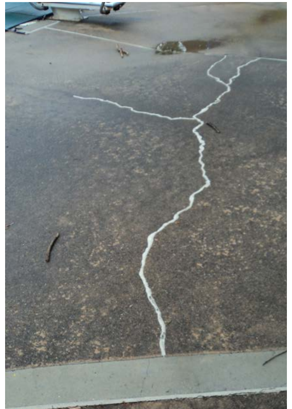
FAILING CONCRETE POOL DECK (T-I-D AND T-II-A)
