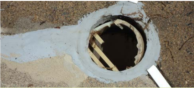
DAMAGED POOL DECK DRAIN (T-I-B AND T-II-B)
