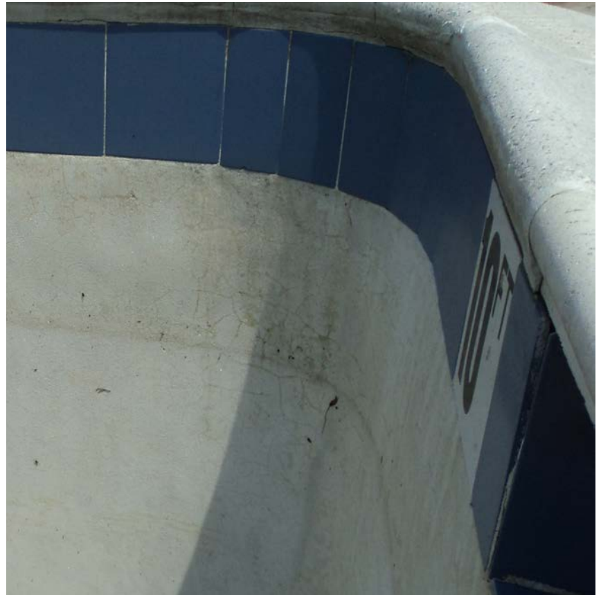
CRACKING / CRAZING IN POOL WALL (T-III-A)
