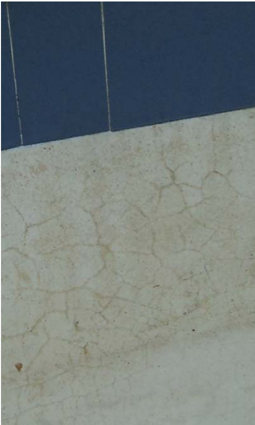
CRACKING / CRAZING IN POOL WALL (T-III-A)
