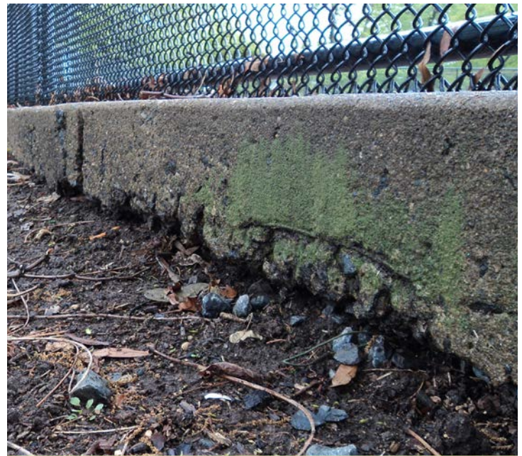
ERODING NORHERN SLOPE AT POOL DECK BASE (T-II-G)
