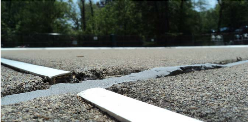
FAILING AND DAMAGED CONCRETE JOINTS (T-I-D)
