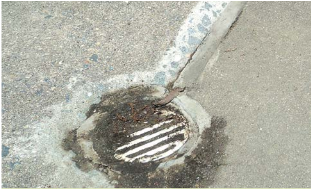
CLOGGED POOL DECK DRAINS (T-I-B)
