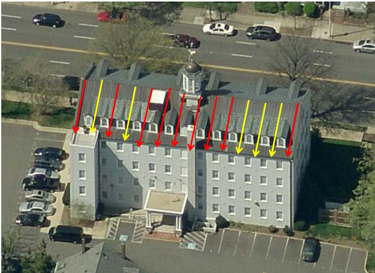
Figure 1. View of rear (east) elevation showing existing dormers. Red arrows indicate roof trusses remaining intact and yellow arrows indicate missing or extensively compromised roof trusses.
