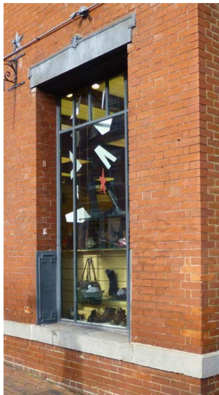
Figure 5. 326 King Street (upper left), 206 South Union Street (upper right), and 201 King Street (above) for modern storefront windows. 201 King Street has a granite sill, significant jamb depth and traditional details including the cast iron lintel, jamb guards and star washers.
