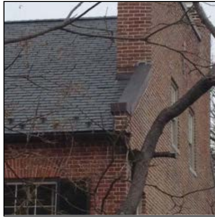
Brick Parapet Termination in Alexandria
