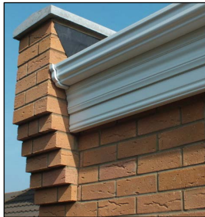
Example of Corbelled Brick Parapet Termination with an Azek Cornice
