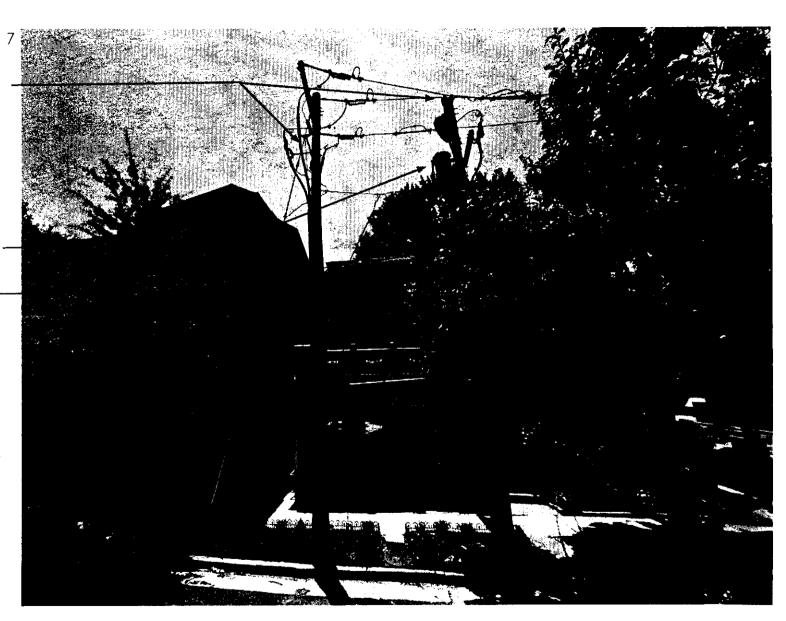
Undergrounding the electrical service requires relocation of the pole mounted transformer to a pad mounted location on the ground
