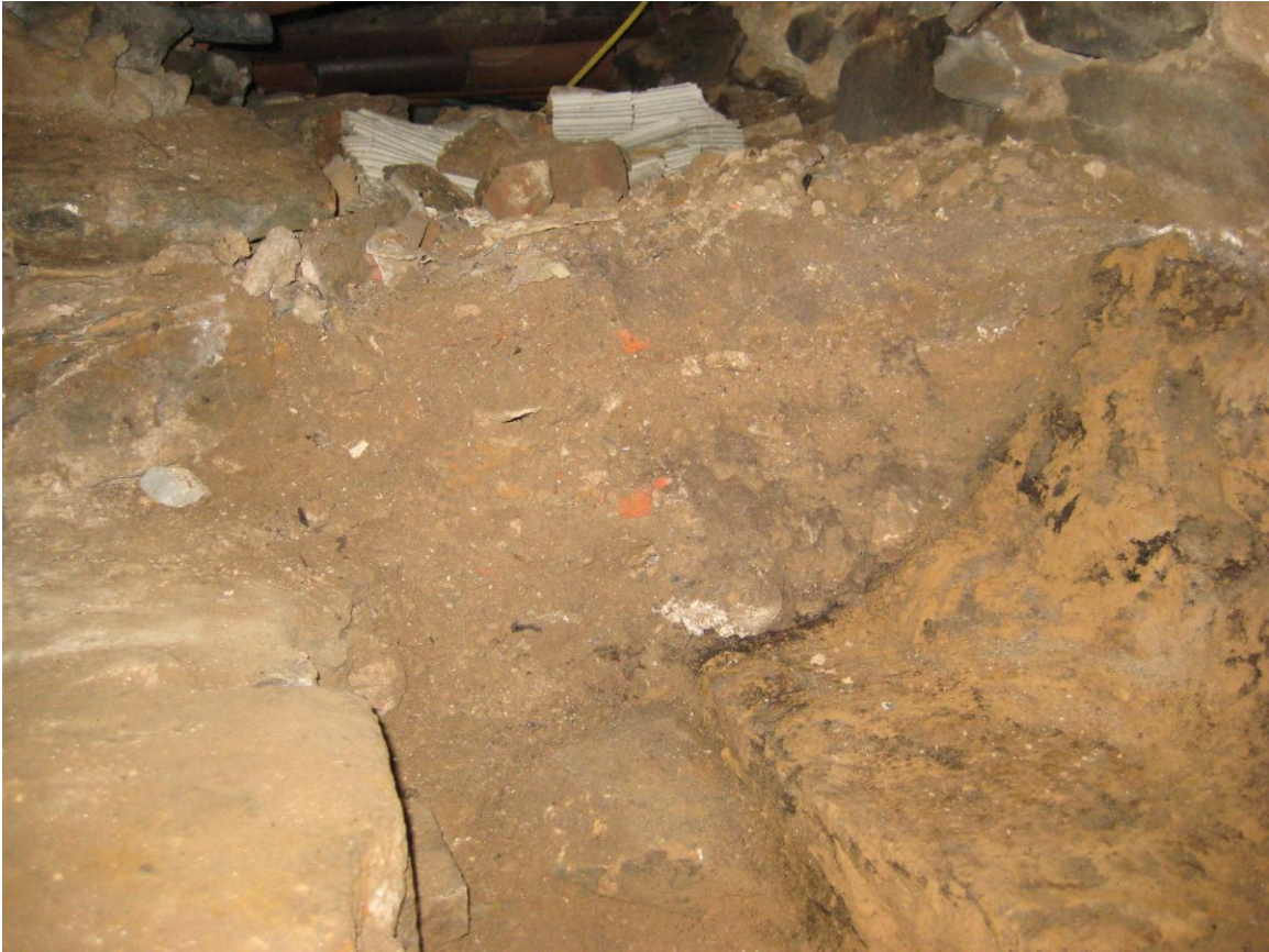
Figure 4. Detail showing the profile of the loose layer of soil and debris overlying the clay subsoil and the builder's trench for the cellar wall.
