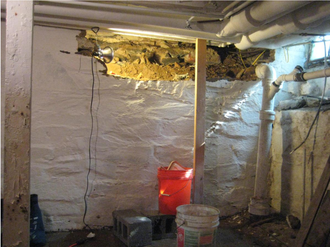
Figure 3. The east portion of the north wall after the top courses of stone were removed to allow access into the crawl space. Note the drain pipe that enters the building at the northeast corner of the north foundation and passes through the cellar.
