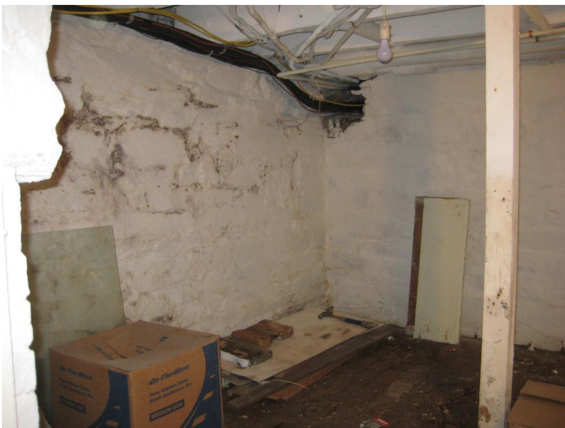
Figure 1. The kitchen cellar, showing the west foundation and the west portion of the north wall. Note the hole in the wall that has been created to accommodate various utility lines, and the relatively smooth character of the wall surfaces.
