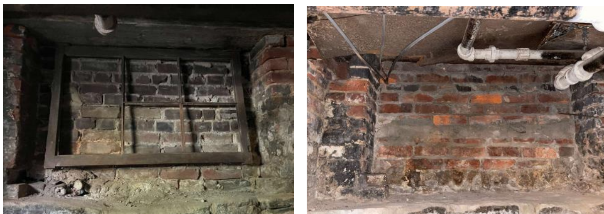
Figure 2: View of previously infilled windows from building interior
