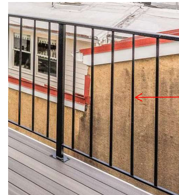
ROOF DECK GUARDRAIL: FABRICATED METAL POST AND TOP RAIL WITH METAL PICKET INFILL
