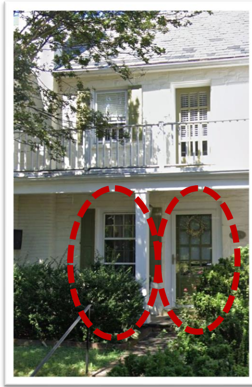
919 S. ST. ASAPH ST. OPERABLE WINDOW DIVIDED LITE FRONT DOOR
