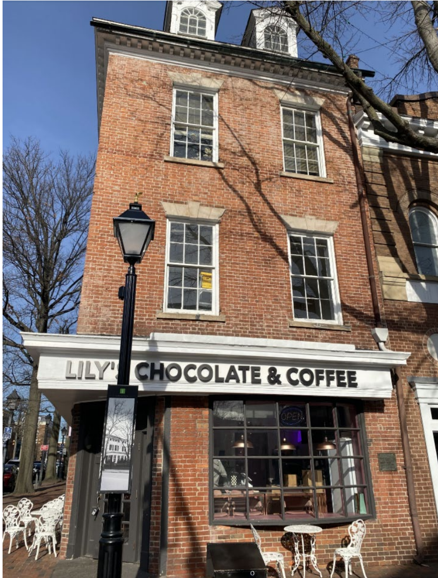
Figure 2: Existing signage at 105 North Washington Street
