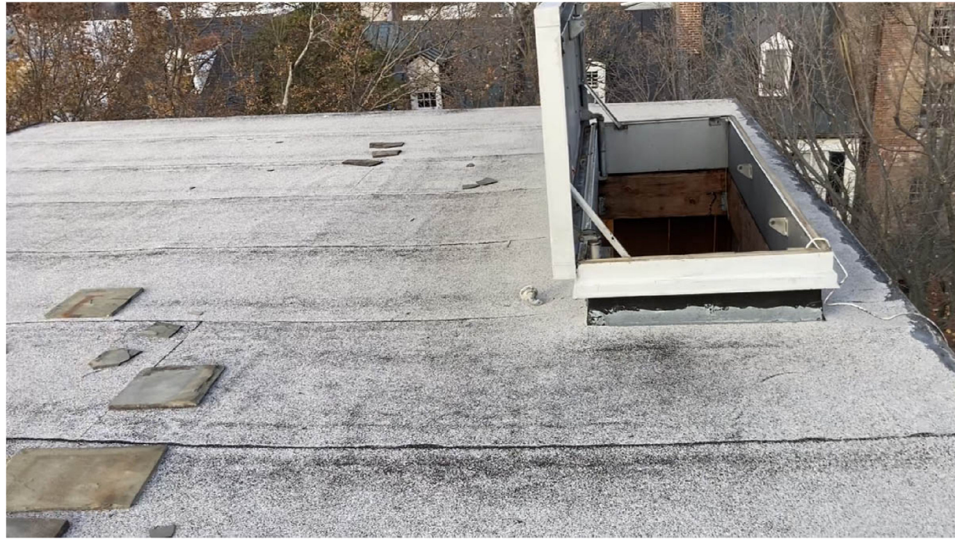
Existing roof hatch looking north
