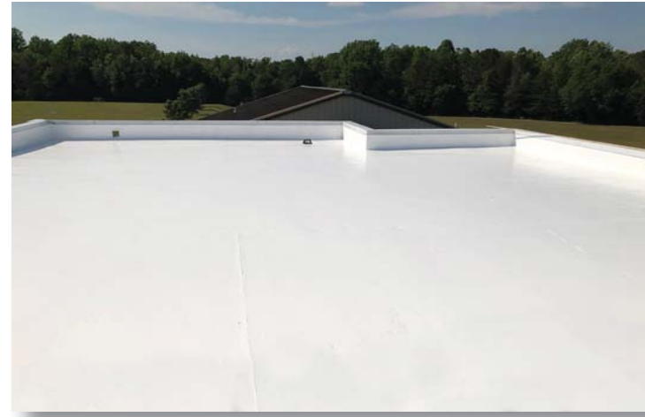
Low slope roof (fluid applied OR TPO (Thermoplastic Polyolefin) membrane color - white
