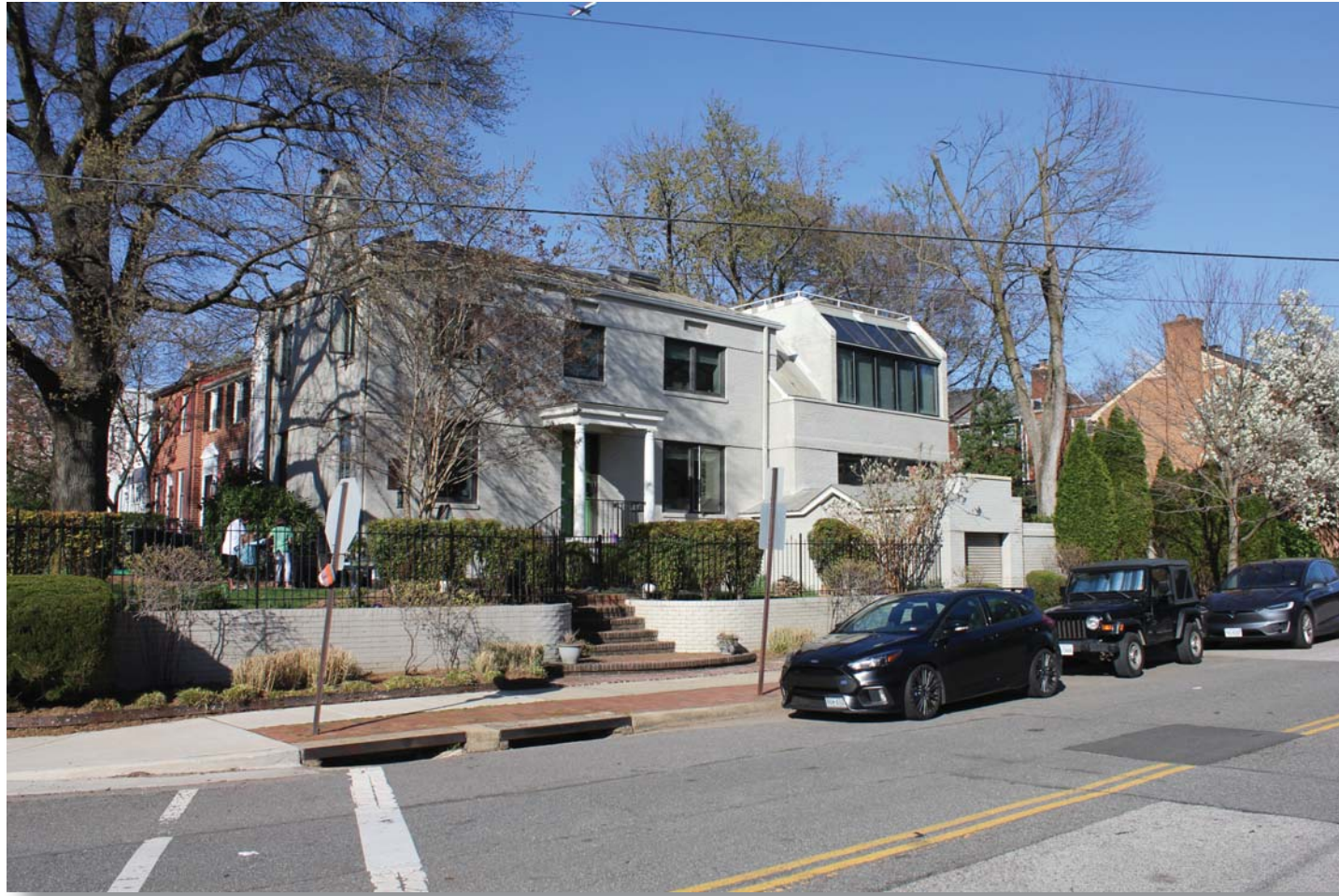
Southwest elevation @ corner of Royal Street & Green Street
