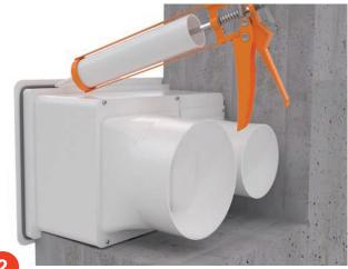
Provide a continuous liberal bead of sealant around rear face flange, as illustrated.
