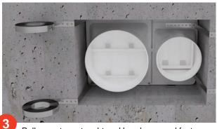
Pull rear straps tought and bend over and fasten with Tapcon or equal.
